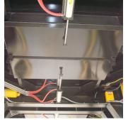
Double clam shell gate doors operated by two air cylinders on ALmix silos. Loss of air load material from the 30 inch silo opening allowing efficient flow and quick loadout.
